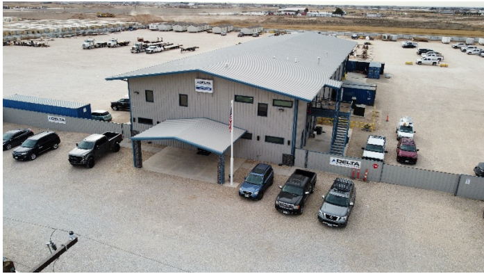
Regional Headquarters Carlsbad, NM
